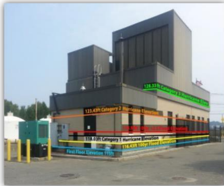
Chelsea Creek Screen House Southwest Facility View
