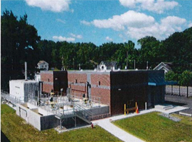
Phosphorus Reduction Facility
