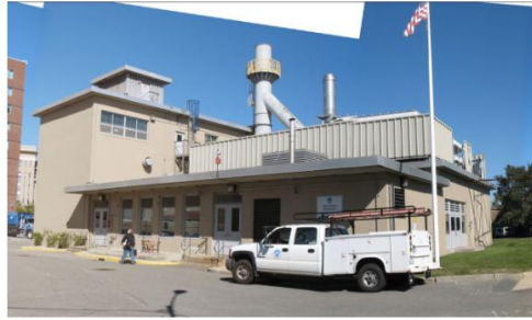
Existing Ward Street Headworks
