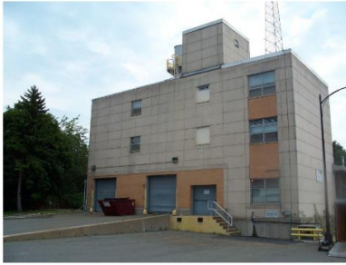
Existing Columbus Park Headworks
