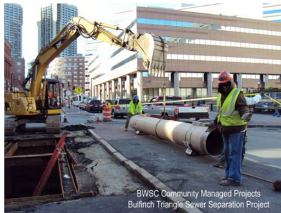
Installation of storm drain on Causeway Street
