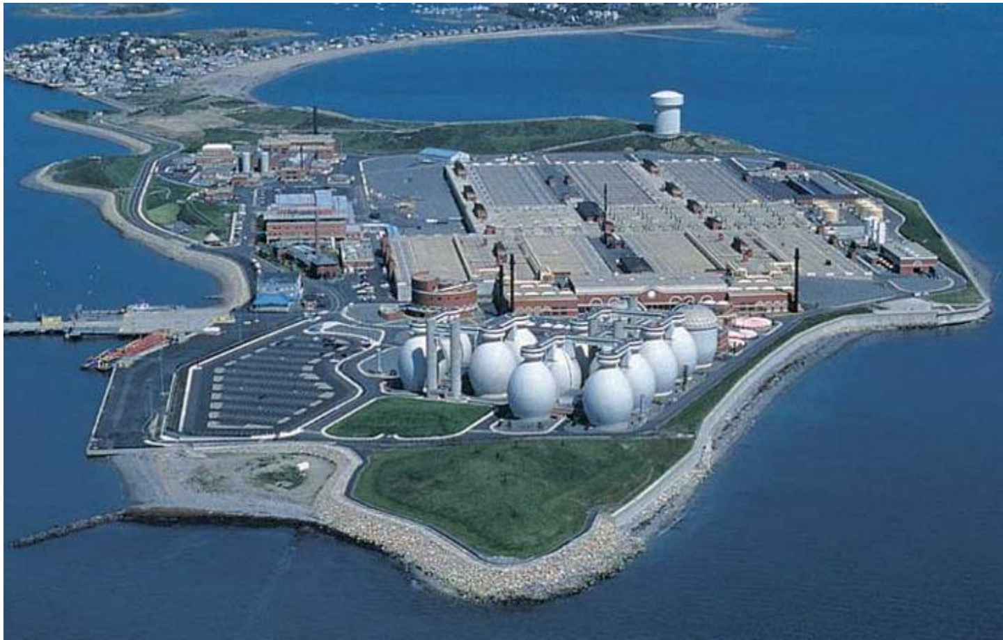
Deer Island Treatment Plant
