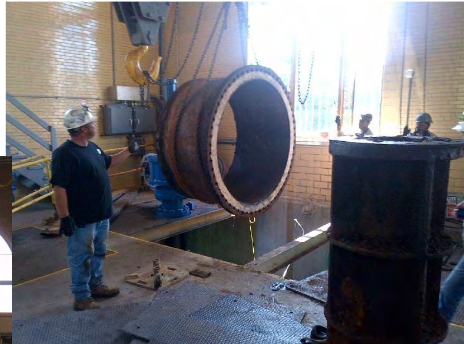
Removing 72-inch Spool Piece
