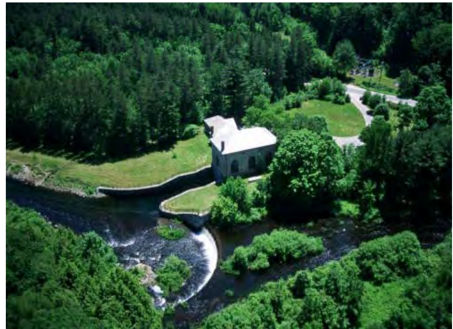
Oakdale Power Facility, West Boylston
