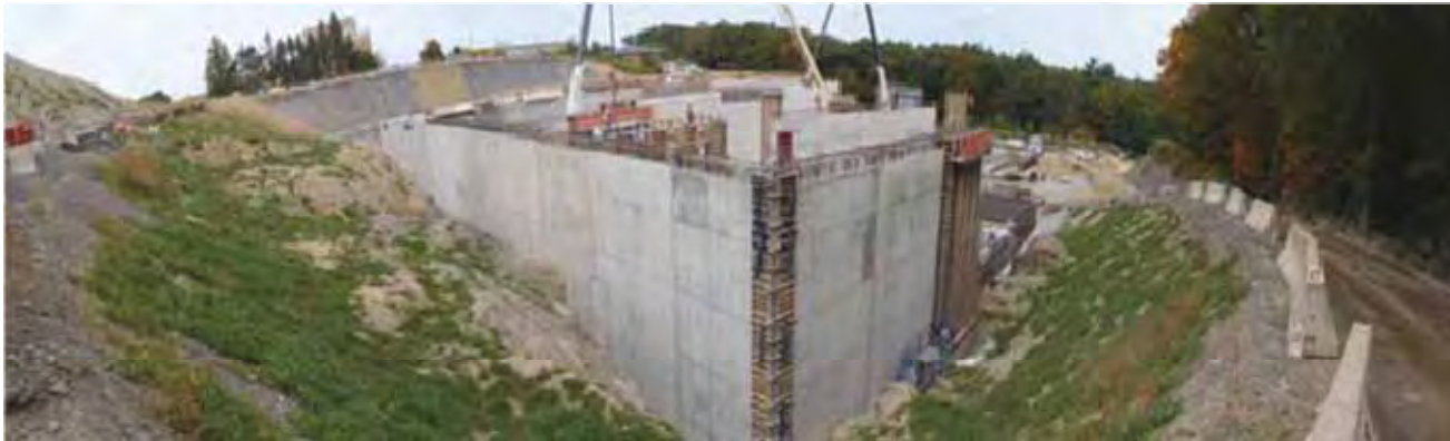
Cell 1 foreground looking north-northwest
