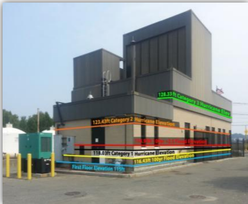
Chelsea Creek Screen House Southwest Facility View
