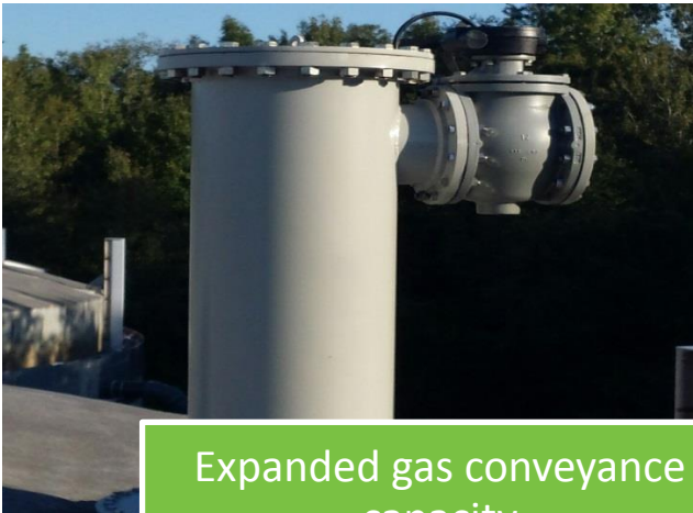
Fixed media (iron sponge) for hydrogen sulfide treatment
