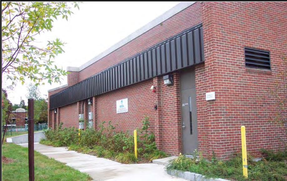
Chlorination and Dechlorination Chemical Building Constructed 2000
