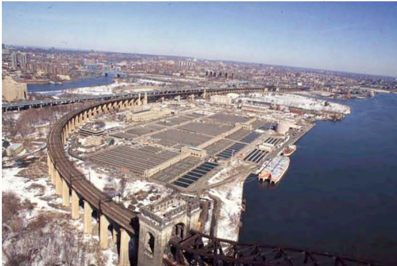
Randall's Island water pollution control plant
