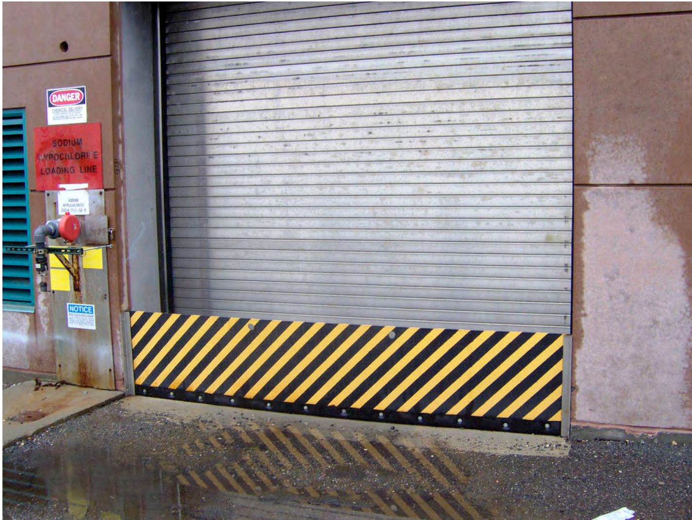
Flood Gate at Tallman Island WPCP
