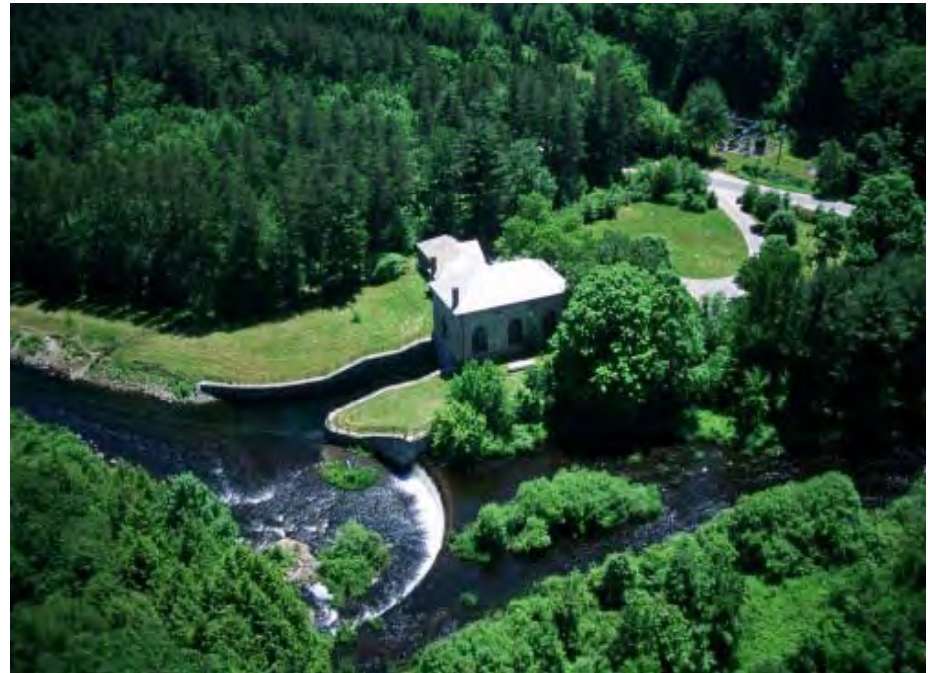
Oakdale Power Facility, West Boylston
