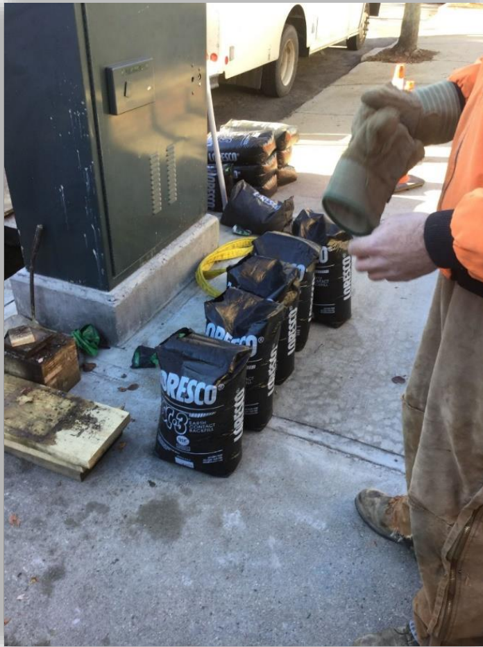
Coke Backfill Material Ready for Placement
