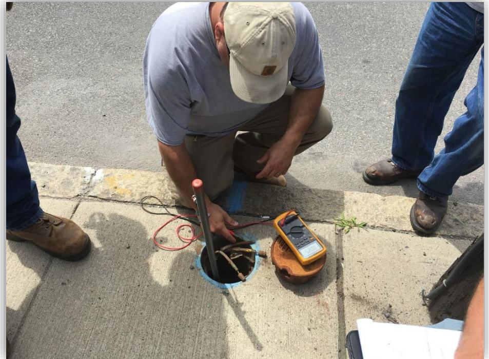
Testing Cathodic Protection Station
