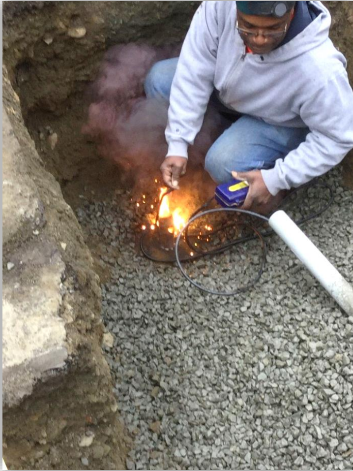
Welding Leads to Pipeline
