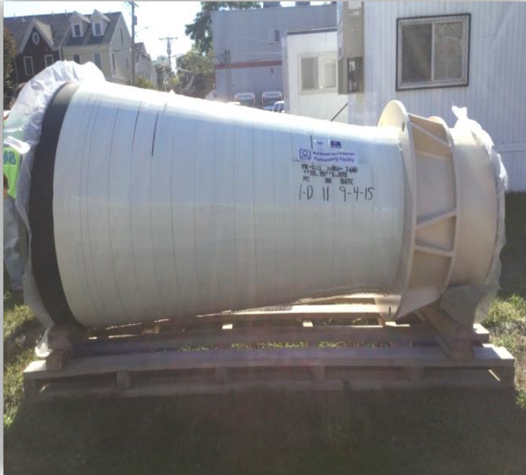
Tape wrapped steel pipe reducer WASM 3 Connection, Arlington
