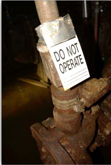
Shaft 8 PRV Chamber
