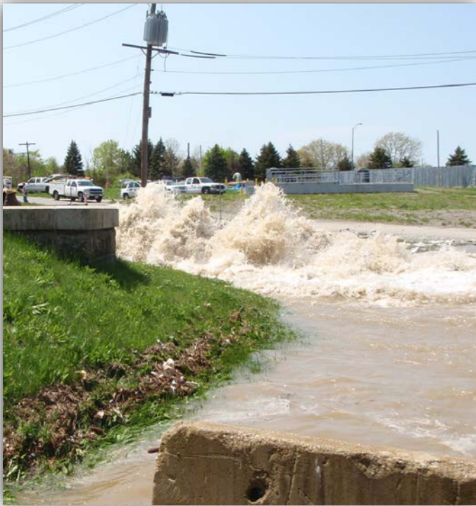
250 MGD flow at Shaft 5 break....
