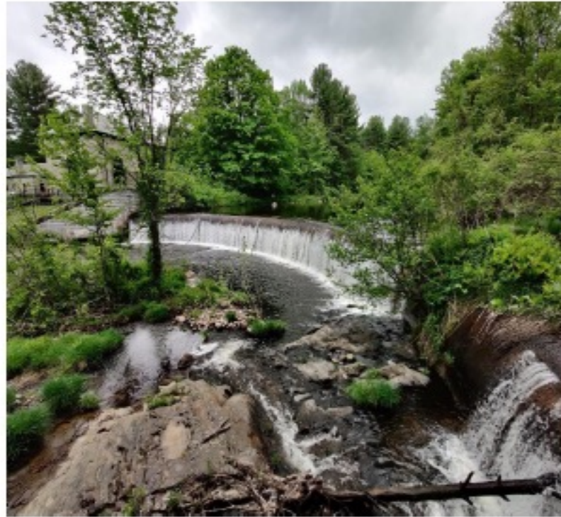
Quinepoint Dam, W. Boylston, MA
