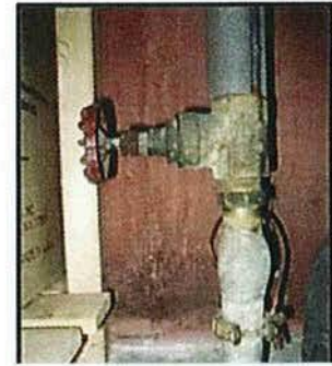
Lead Service Line Entering Basement
