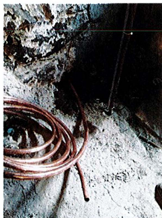
Replacement of Lead Water Services with Copper Service Pipe
