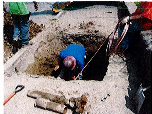
Replacement of Lead Water Services with Copper Service Pipe
