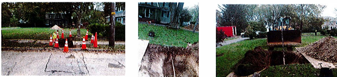
Long lead service line replacement in Newton
