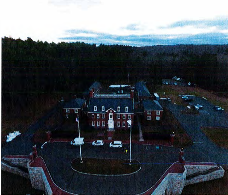
Figure 2: Quabbin Administration Building
