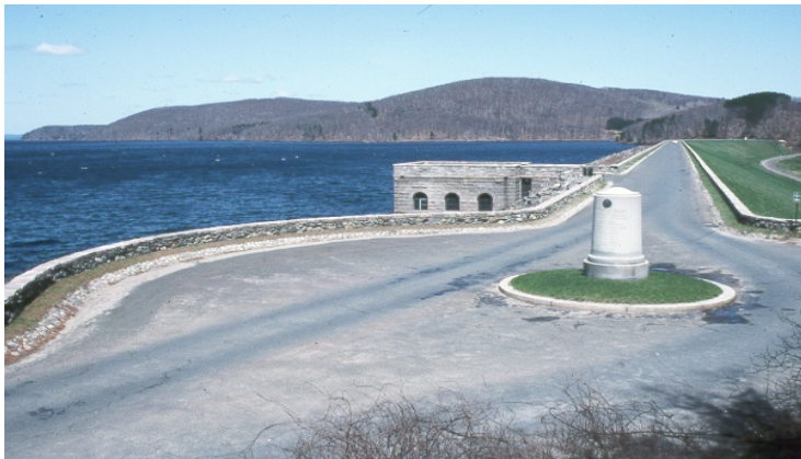
Winsor Dam at the Quabbin Reservoir
