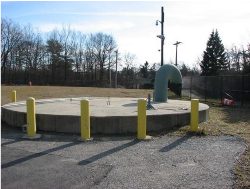
Figure 4.4-4 Top of Shaft Structure Metrowest Water Supply Tunnel, Weston
