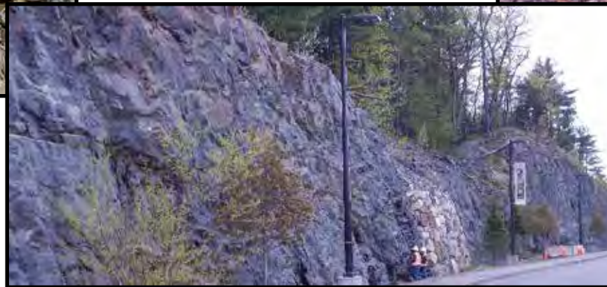
Roadway rock cut on Border Rd in Waltham
