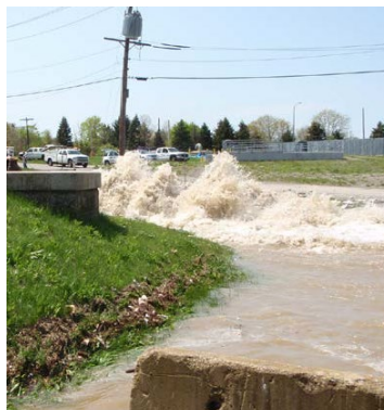
Figure 1.4: The Great Water Main Break of May 2010
