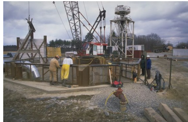
Example of shaft construction activity
