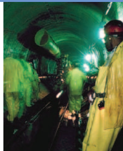
MetroWest Water Supply Tunnel groundbreaking
