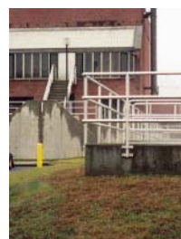
Clinton Wastewater Treatment Plant completed
