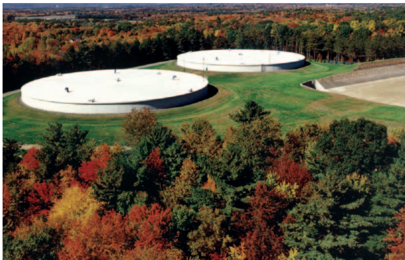
Nash Hill Covered Storage Tanks
