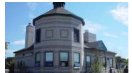
Hultman Aqueduct and Norumbega Reservoir were taken off line
