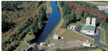
Interim Corrosion Control Facility in Marlborough completed
