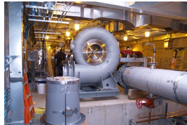
Loring Road Hydroelectric Generator during construction
