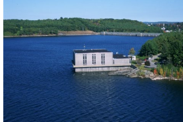
Hydroelectric generators at the Cosgrove Intake capture energy as water leaves the Wachusett Reservoir headed toward metropolitan Boston area.
