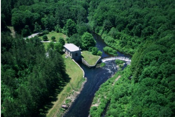
The Oakdale Hydroelectric Generation facility captures energy as water enters the Wachusett Reservoir from the Quabbin Reservoir.
