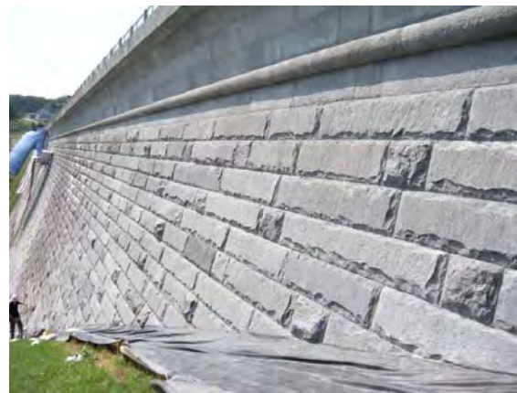
Wachusett Dam, post PCB remediation, repointing and cleaning
