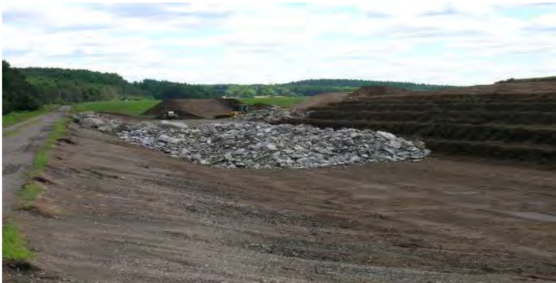
North Dike structural improvements
