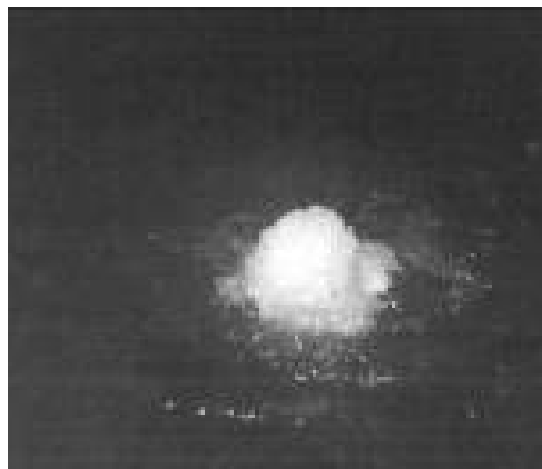
Leak Boil in Floor
