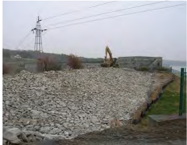
East Berm armored
