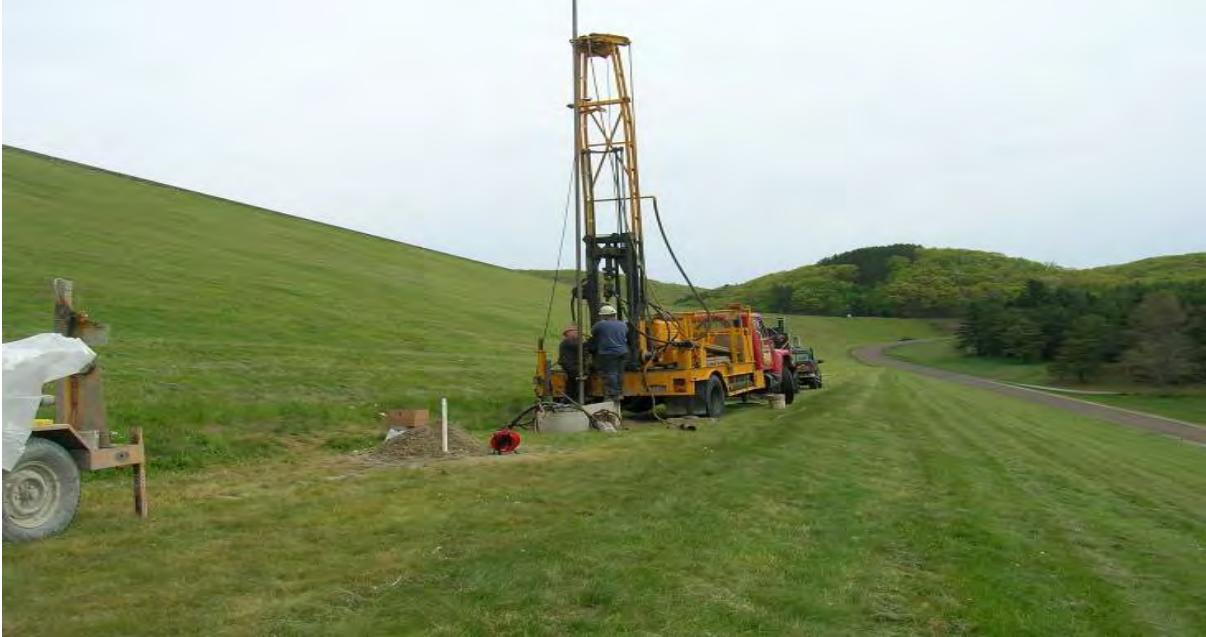
Piezometer installation at Winsor Dam
