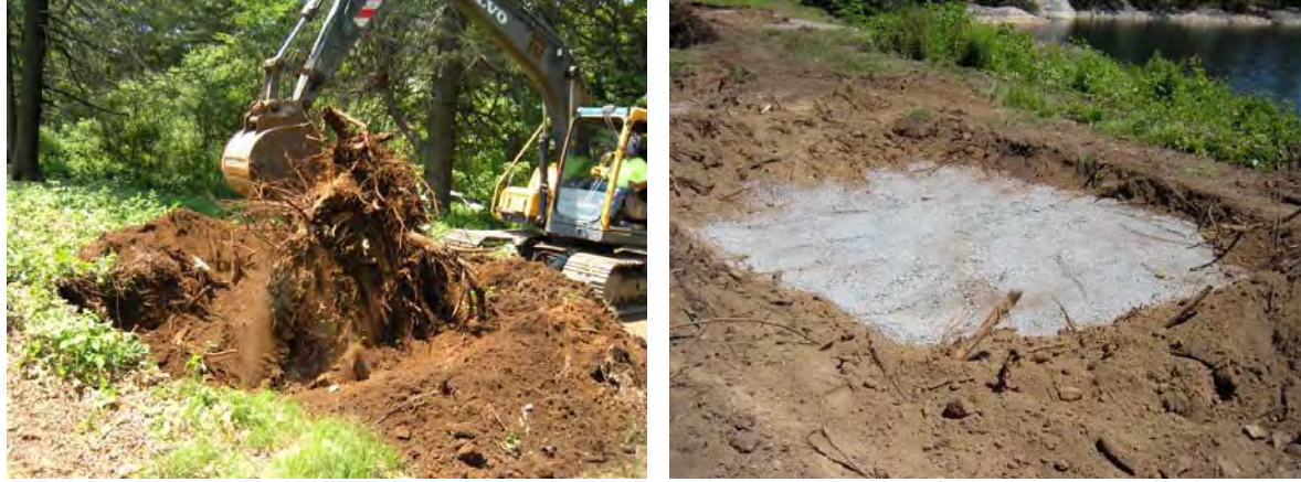
Stump removal from dam
