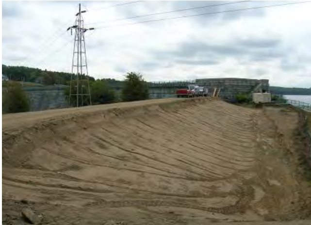
East Berm created along left abutment
