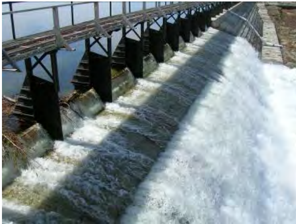
Old stop log bays, sill at 392' BCB
