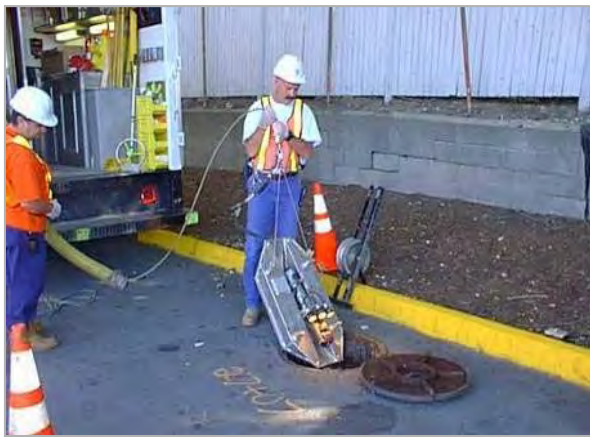
CCTV Inspection Crew
