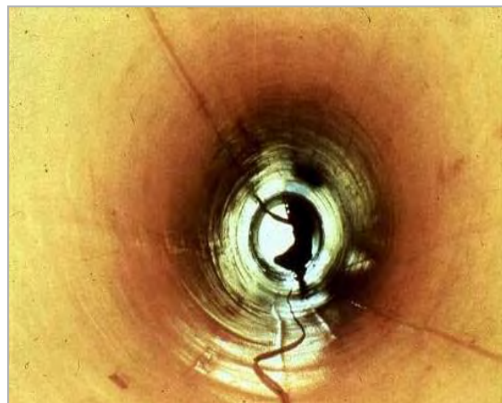
Example of sewer rehabilitated with cured-in-place pipe (CIPP) liner
