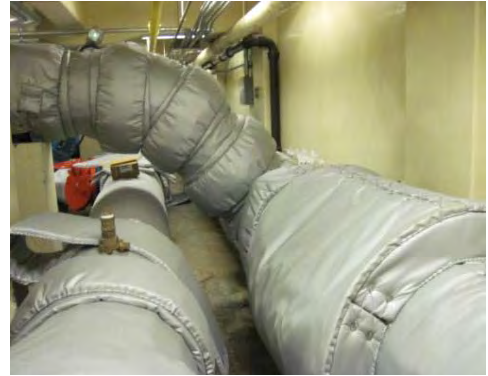
Insulation of Water Piping
