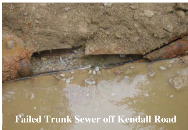
Excavation of Kendall Road Trunk Sewer
