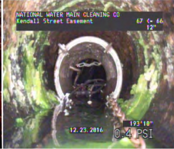
Injection Grouting Repair
