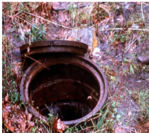
Inflow into a sewer manhole located in a ponded wetland area
