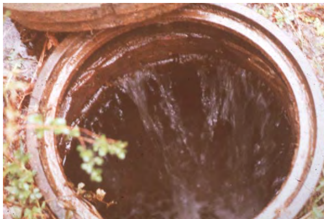
Inflow into a sewer manhole located in a ponded wetland area
