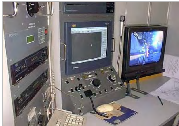
Inside of CCTV Inspection Truck
