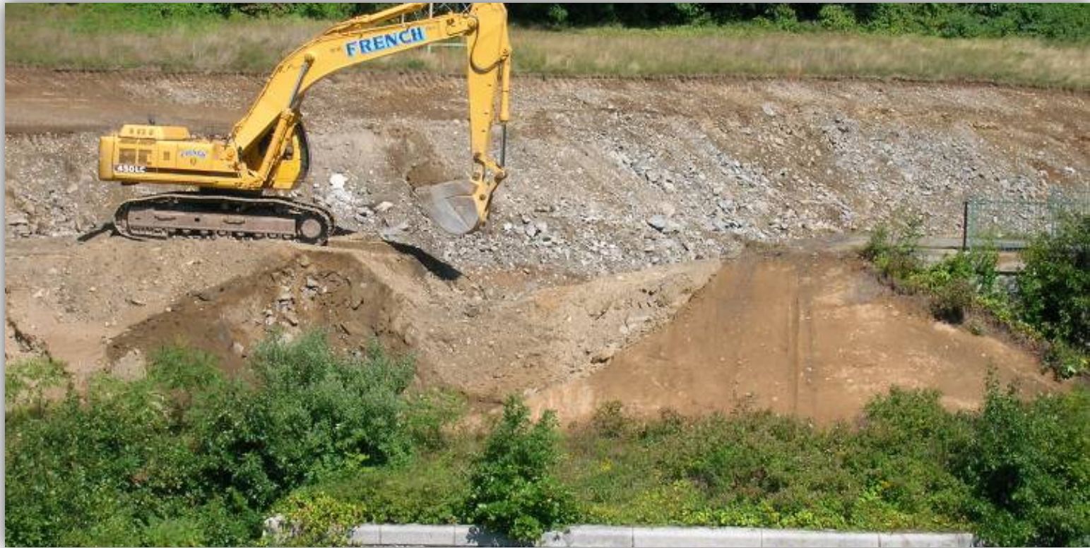
New Wachusett Auxiliary Spillway constructed to pass flood discharge
