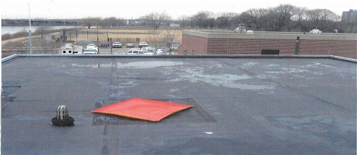
**Rooftop Drain where Fuel Oil Leaked through Internal Piping to Charles River**
