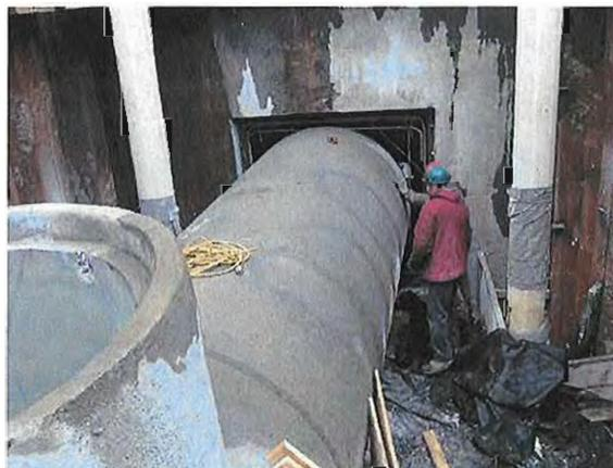
New 60-inch PCCP pipe interconnection between the North & South Charles Relief Sewer overflow chambers in the Cottage Farm yard.
