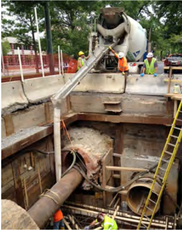
Special Structure 6, Beacon Street, Brookline, June 2012
