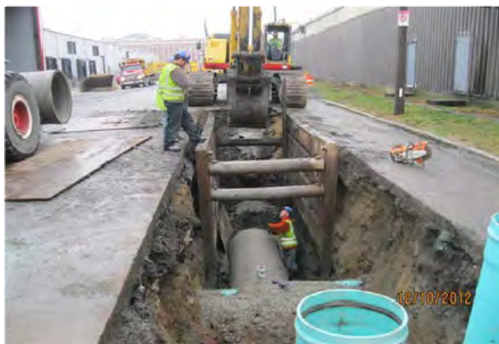
Installation of 36-inch Storm Drain on E St. (Contract 4)
