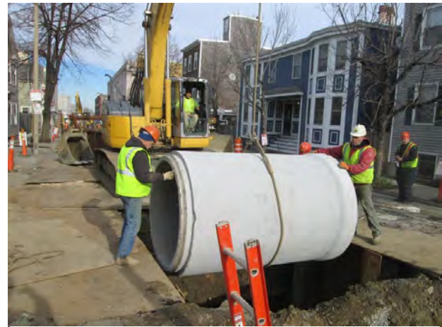
Installation of 54-inch Storm Drain on K St., South Boston
