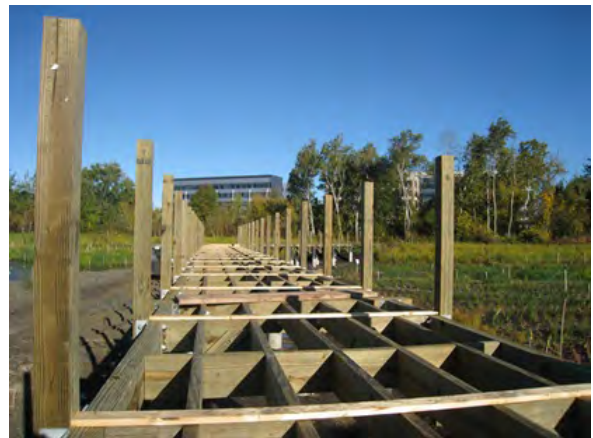
Framing of Boardwalk across Main Basin, October 2012
