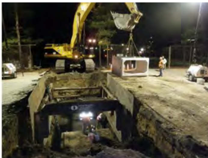
Nighttime Construction of Stormwater Box Conduit on Upper Wheeler Street, February 2012
