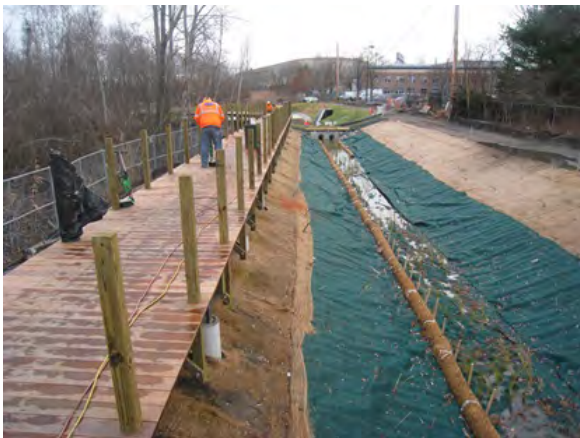
Construction of Boardwalk and Vegetated Swale from Forebay to Main Wetland Basin, December 2012
