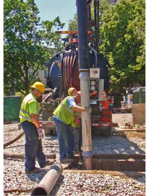
Contractor removing sediment from CSO Outfall MWR010
