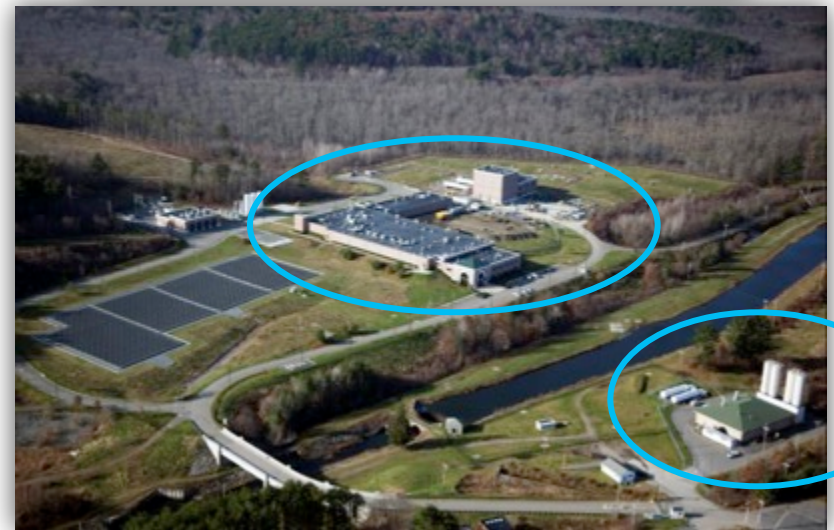
The John J Carroll Water Treatment Plant (center) and Interim Corrosion Control Facility (foreground) provide continuous corrosion control treatment since 1996
